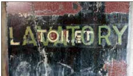
*The original varnished wood finish and lettering have been exposed beneath the maroon coloured paint on this toilet door. This panel is preserved and has been reinstated on the door into the store from the corridor. It has been reversed so that this side faces the store room.*
