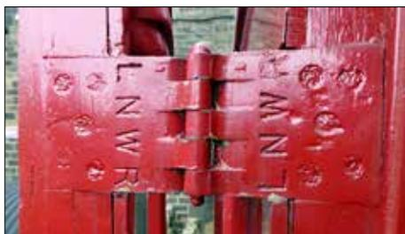
*The top hinge of one of the compartment side doors indicating how such standard features were utilised in different eras.*
