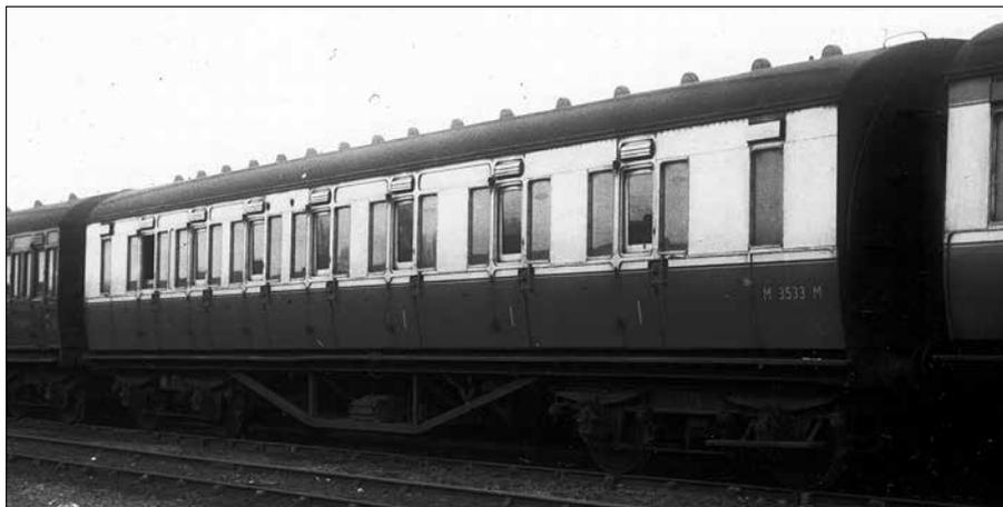
*Withdrawn from service in May 1958, this 57ft corridor composite coach, No.M3533M, in its crimson and cream livery, is awaiting conversion in to a Riding & Tool Van at Wolverton. Completed in the same period as No.3515, this vehicle became DM 395478, part of the breakdown train at Westhouses motive power depot in Derbyshire. photo: R M Casserley*
